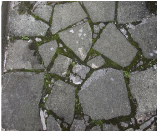
Fig. 7.8 Craze paving as an illustration of a hybrid resin-based composite. The differing sizes and shapes of the stones (filler particles) reduce the amount of cement (resin) as they are able to pack more closely together.
