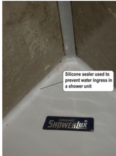
Fig. 15.23 A silicone material used to seal around a shower to contain water within the shower unit.
